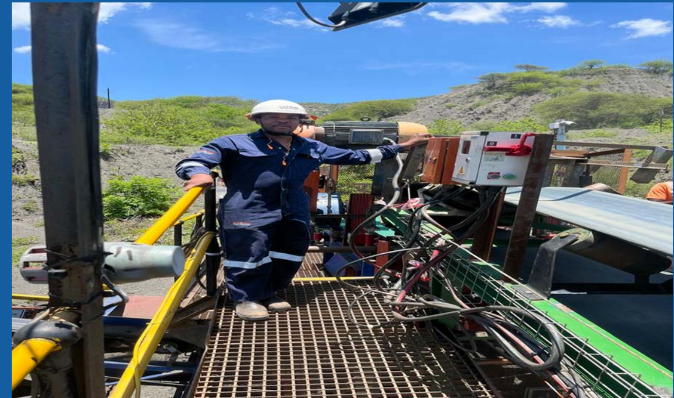
Maintenance of conveyor belt systems
